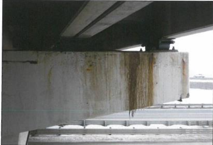
9. North end of pier 3 icing, corrosion stains, cracks at girder 8/9 bearing area.
