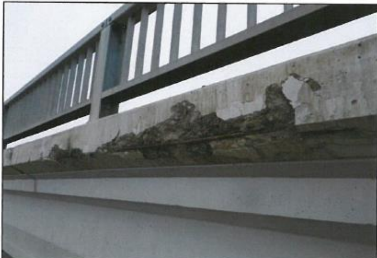
10. Span 4 south curb spalling, exposing rebar.
