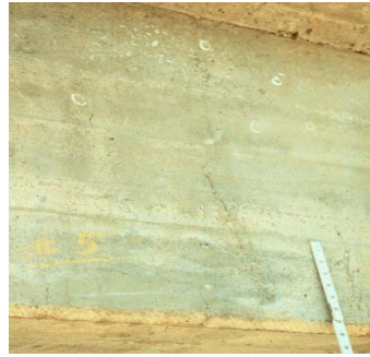
(b) Flexural crack on a tee beam
