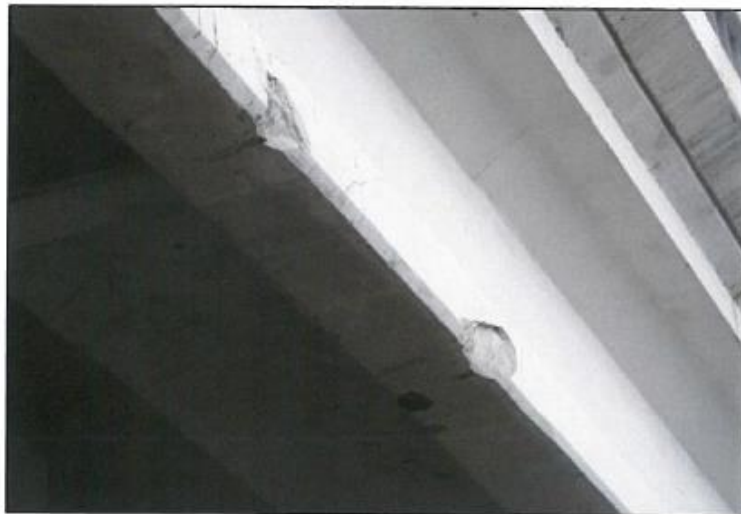
16. High load chips to span 2 girder 1 over outside lane.
