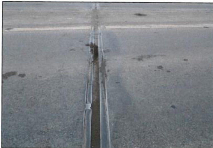
12. Missing plow guards, ripped gland at pier 3 gland WBL.
