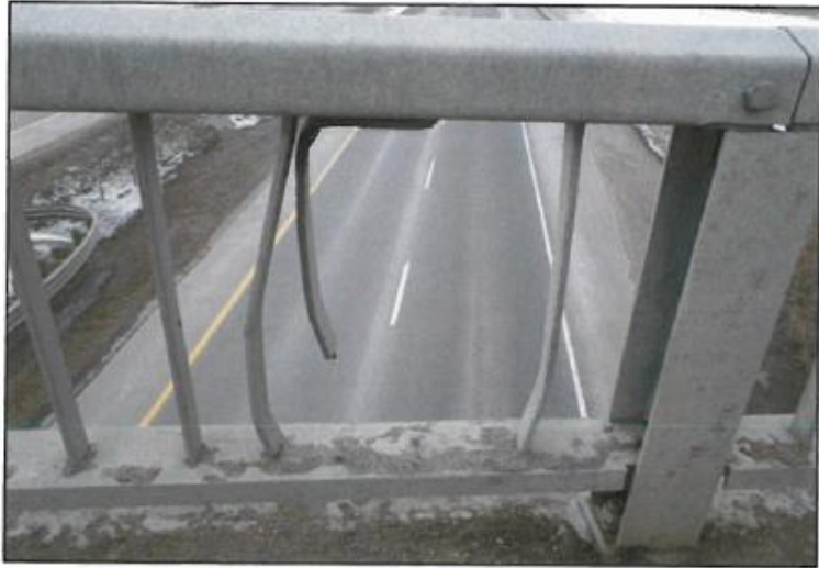
13. Damaged rail panel, 7th panel from SW.
