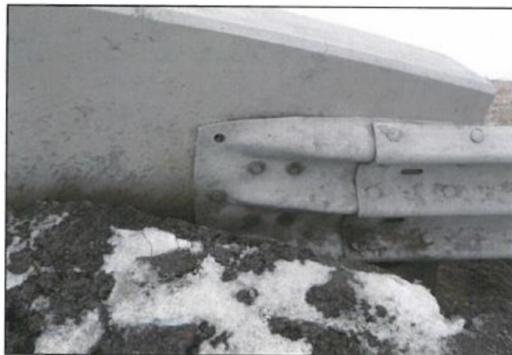
14. Missing SW transition connection bolt.
