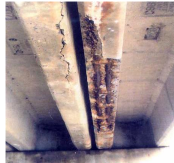
(e) Spalling on leg of curb girder
