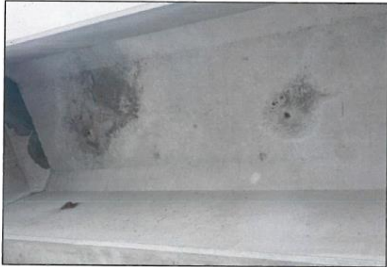
5. Span 4 girder 1 scale at weep drains - typical.
