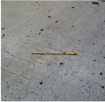
(a) Shrinkage cracks on a deck
