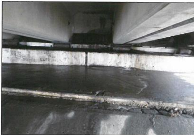
6. SE slope protection icing on bearing seat. Gap at top of east slope protection.
