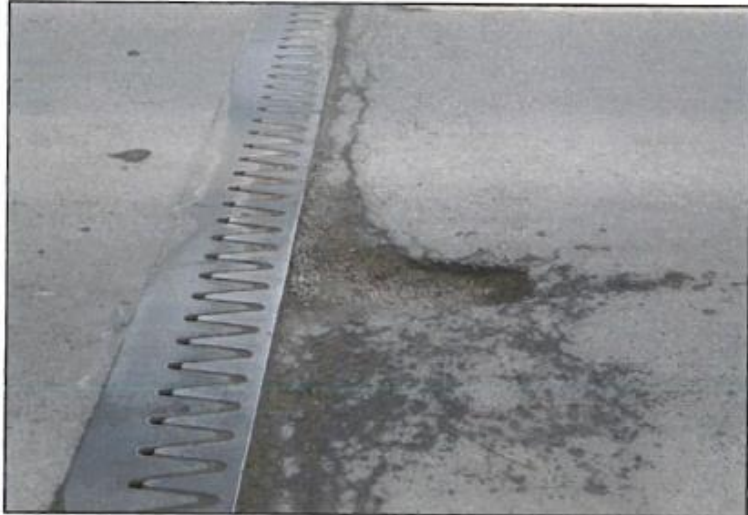
11. Wheel path pothole at abut 2 joint, EBL.
