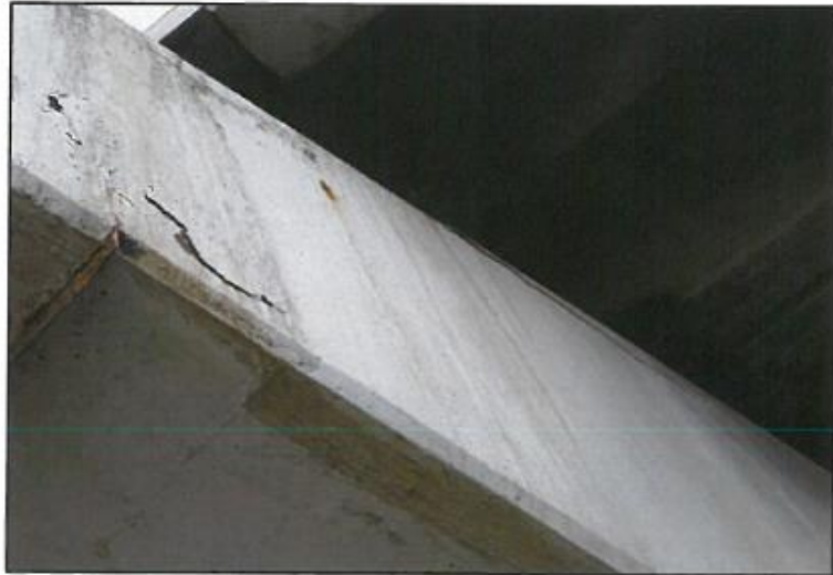
17. South end pier 1 minor delamination at drip guard, cracking near bearing.
