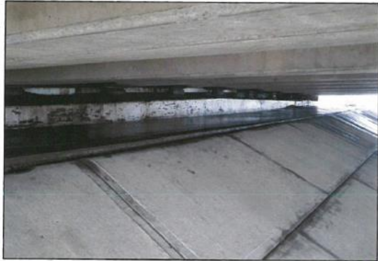
15. Icing at abut 1 slope protection, gap at bench, typical bearing seat sealant condition.
