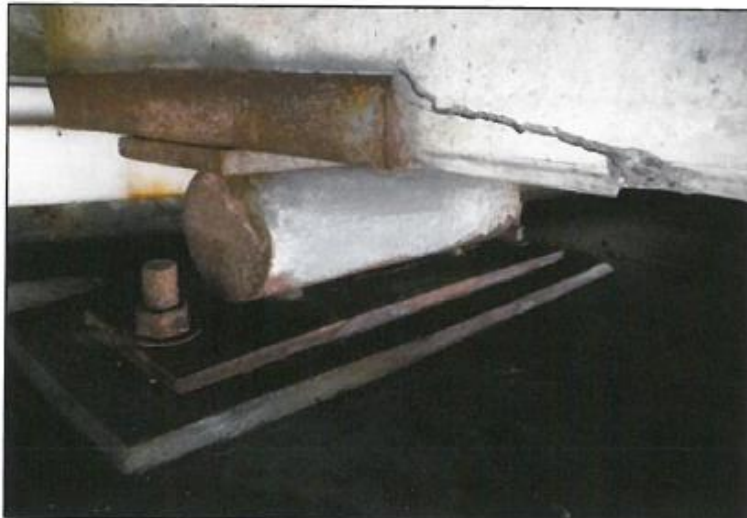
8. Span 4 girder 4 wide shoe crack, typical roller condition.
