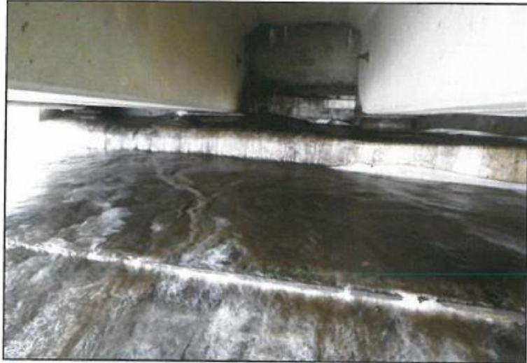
7. Icing at NE bearing seat and slope protection.
