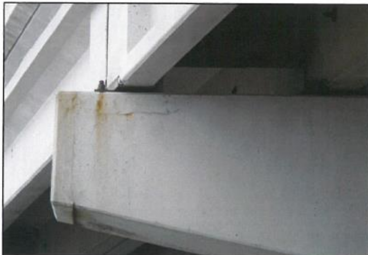
18. Pier 2 north end cracked on west face.
