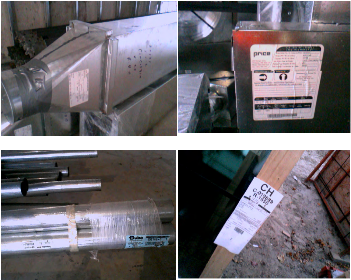
Figure 4-17: Items with barcode inside Genomics building jobsite
