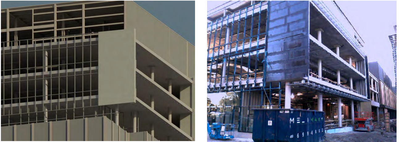
Figure 4-15: 4D BIM image vs. actual image for outdoor zone
