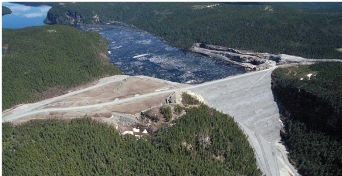
Figure 4-20: Sainte-Marguerite-3 dam (Hydro Quebec 2003)
