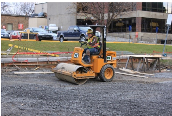
(a) During Compaction Process
