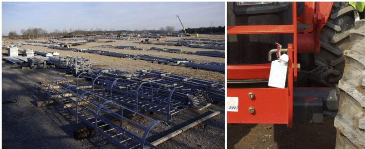
Figure 2.9 – UWB Tracking in Lay Down Yard (Saidi et al., 2011)
