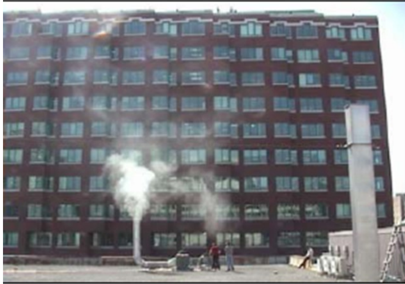
Figure 2-4. Roof of BE building, Concordia University, Montreal
