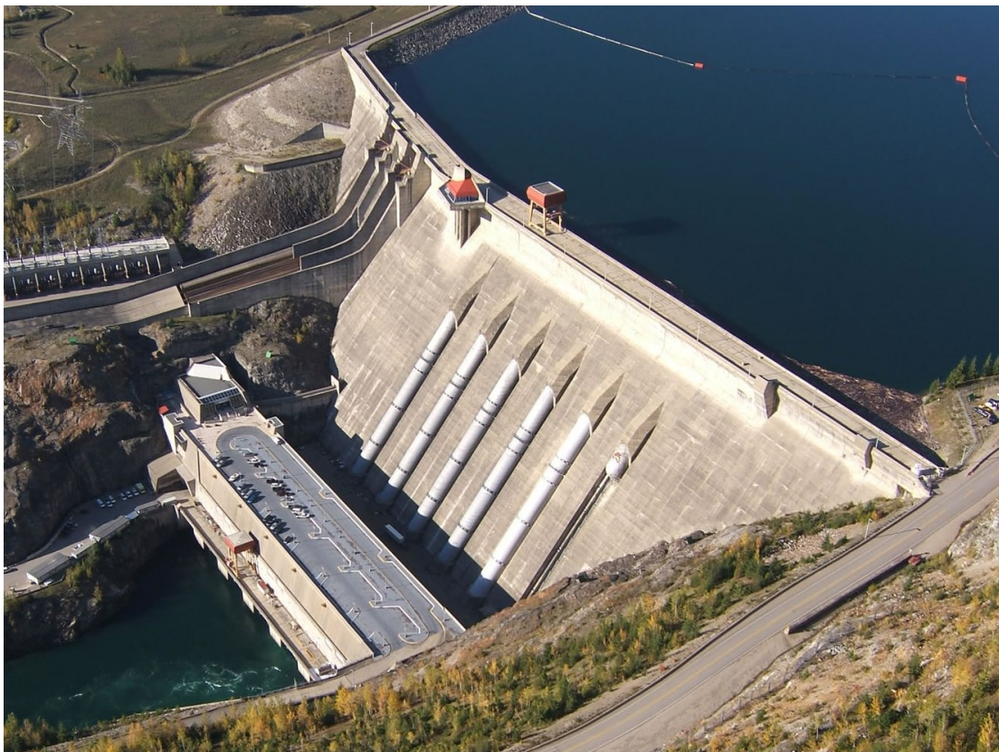
Figure 3-6 An aerial view of the Revelstoke Dam in British Columbia. Five penstocks are shown to hug the slope side of the dam (adopted from B.C. Hydro).
