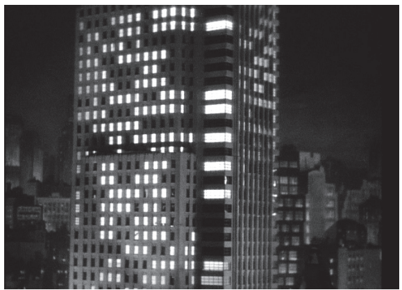
Figure 1.11 The Baldwin Building completed.
