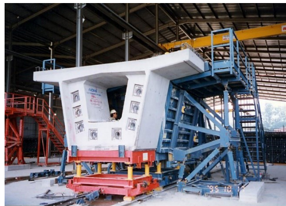
(b) Short line casting method
