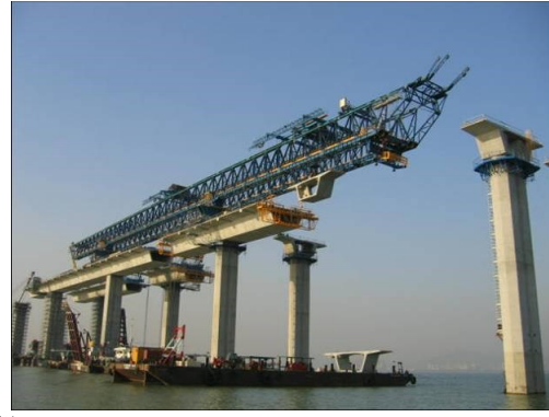
(b) Balanced cantilever erection with launching gantry
