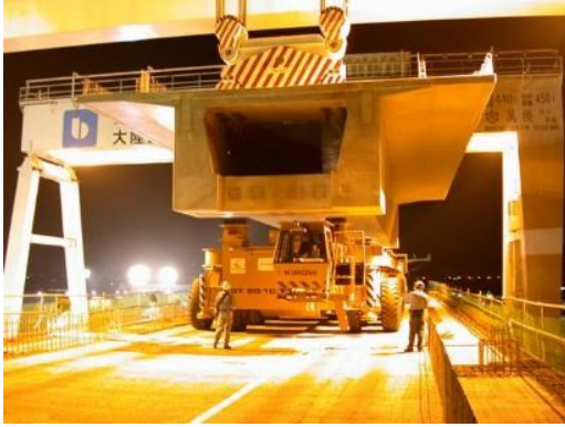
(a) Transporting precast full-span to the main site
