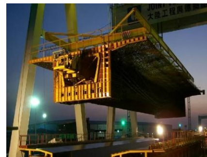
(c) Putting rebar cage into outer mold
