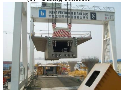
(h) Transporting completed span to the storage area
