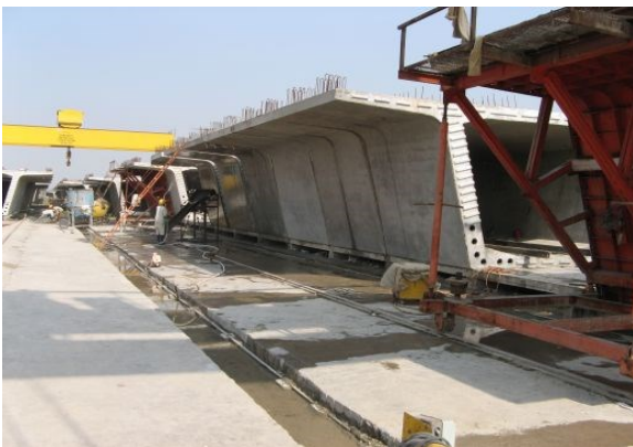
(a) Long line casting method
