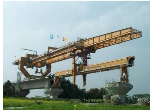
(f) Reposition launcher to the next span
