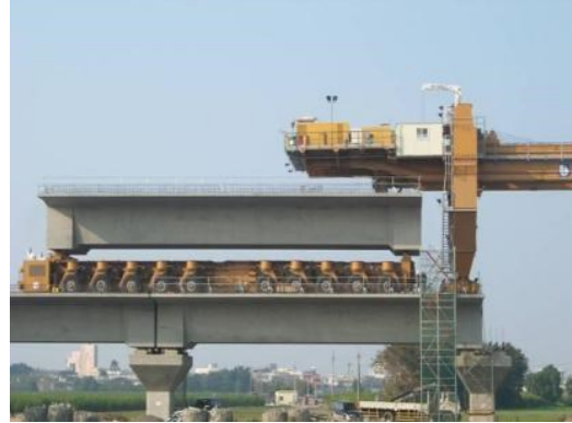
(b) Delivering the girder to the launcher by trolley
