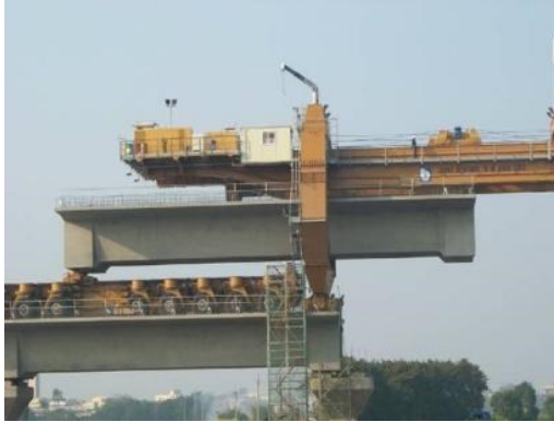
(c) Lifting the girder by lifting frame
