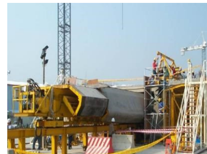
(f) Removing inner mold
