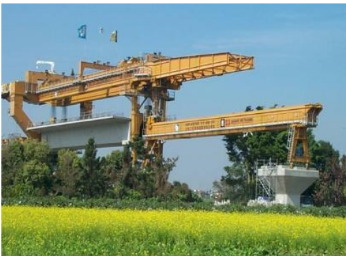
(e) Locating the span in its right position
