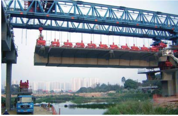
(a) Span by span erection with launching gantry
