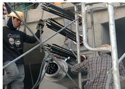
(g) First stage of pre-stressing
