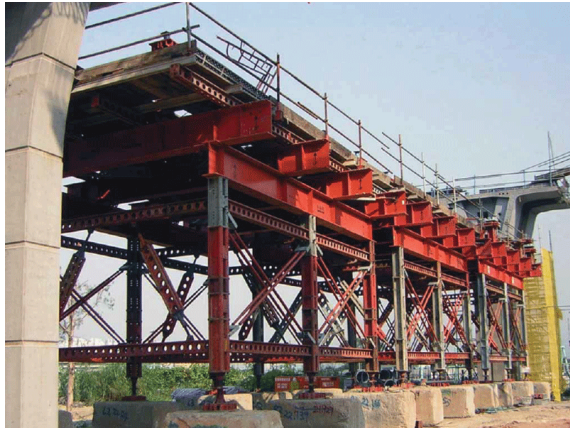
(c) Span by span erection with false-work
