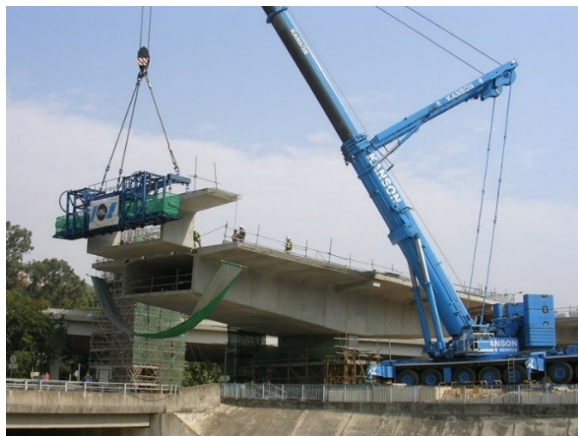
(e) Balanced cantilever erection with cranes
