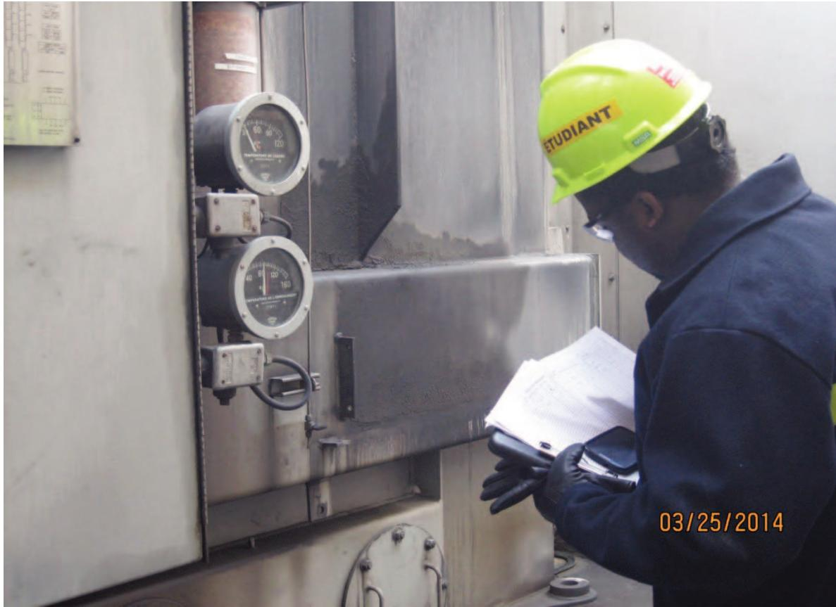
Figure A.14 Alcoa Rectifier Transformer TR43 Top Oil and Hotspot Temperature Guages
