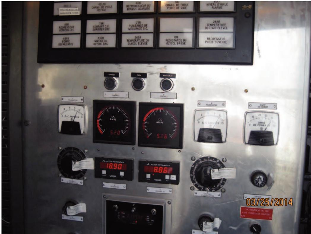
Figure A.13 Alcoa Rectifier Transformer TR43 Output DC Current Panel
