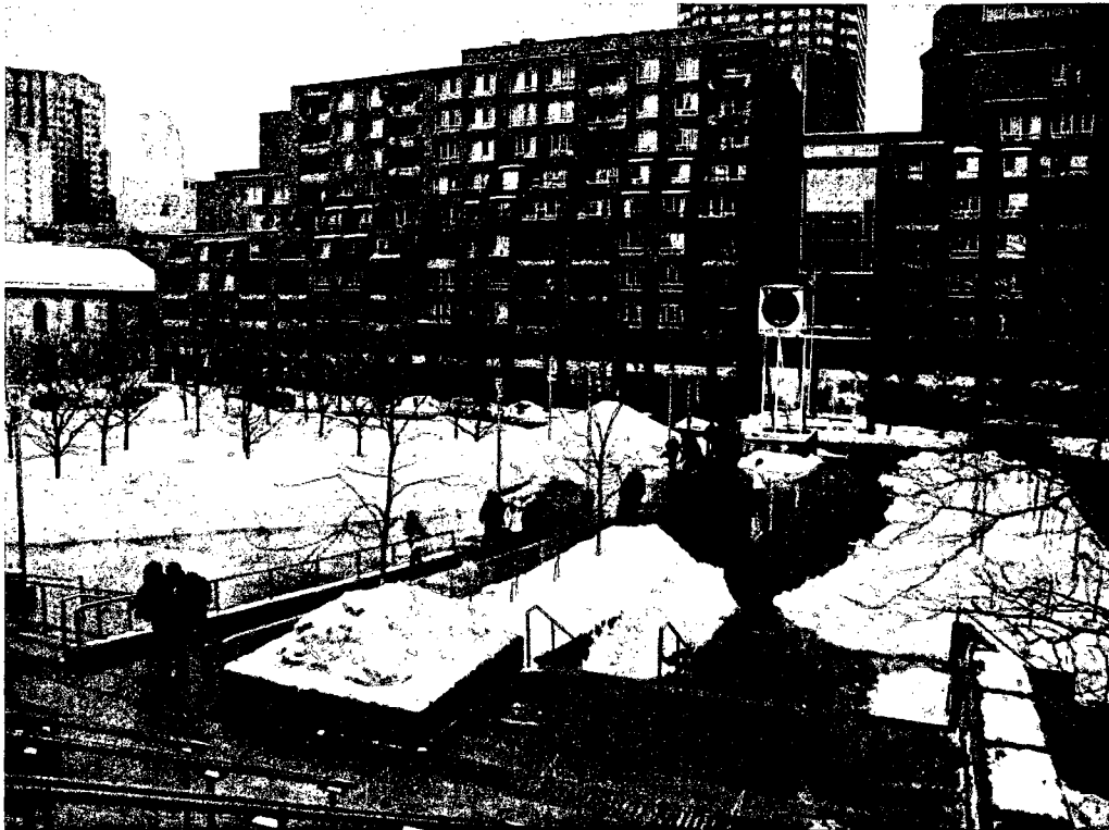
Figure 1.4-13: Complexe Guy-Favreau building
