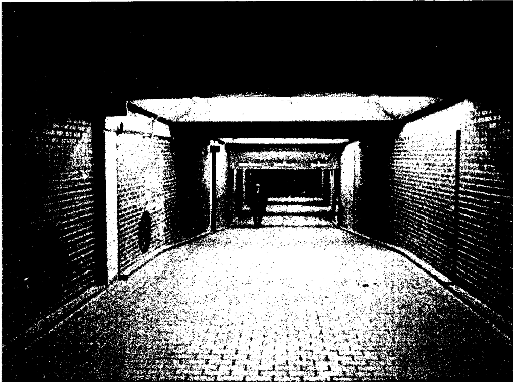
Figure 1.4-15: Interior view of tunnel #3
