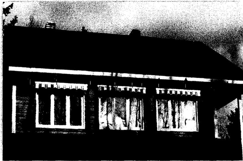
Figure 3.2. Photograph of the BIPV/T roof in the EcoTerra™ House. The amorphous PV modules are attached to a metal roof skin on vertical and horizontal wood framing that also creates the flow channel. (The roof has a length of 5.8 m in the flow direction shown by the arrows).
