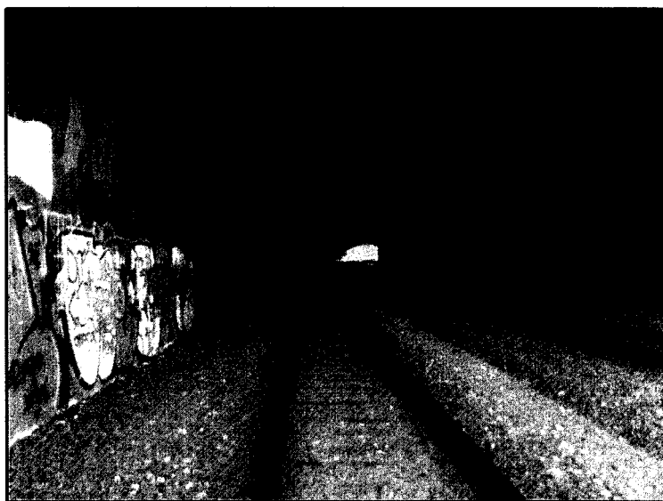
Figure 2.7 Inside walls of Turcot train tunnel, April 2009
