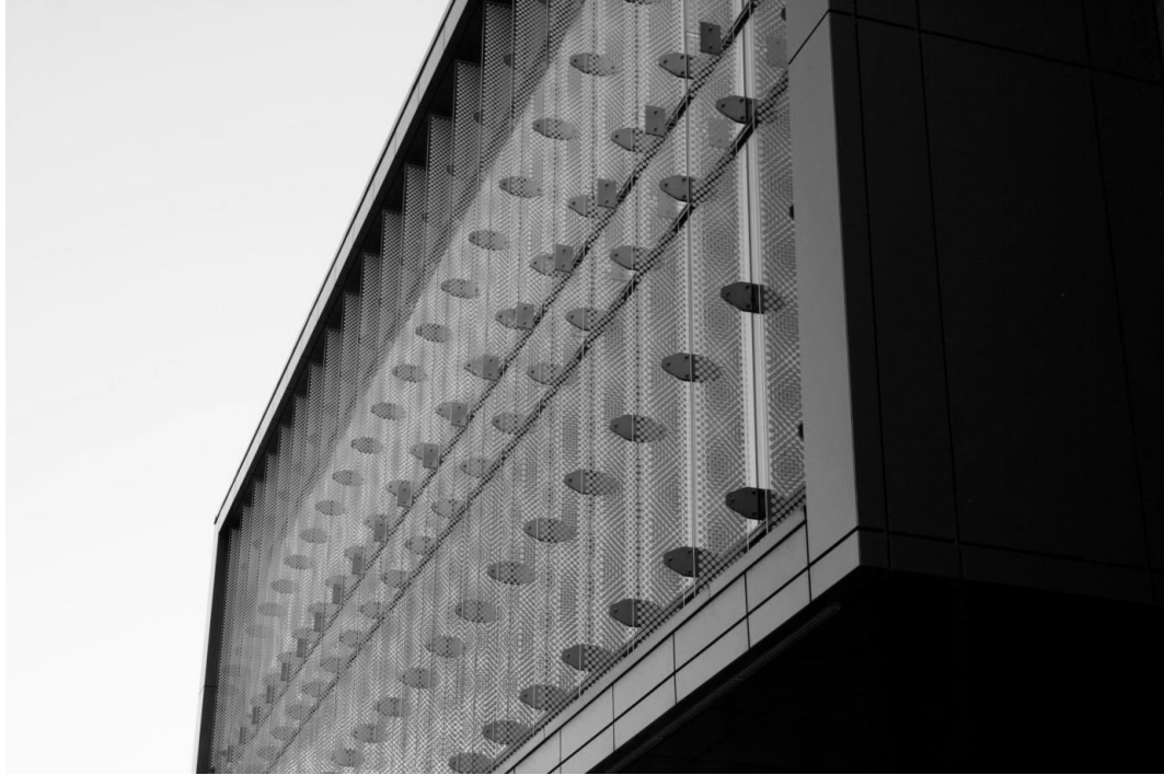
Figure 3.6 Fritted vertical fins on the northeast surface
