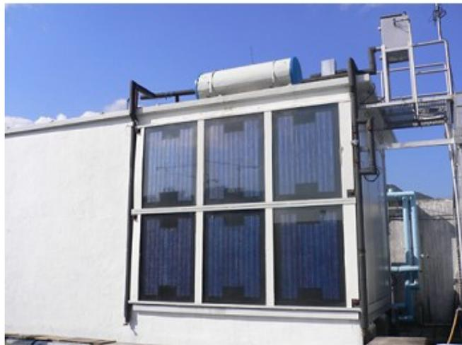
Figure 2.18. A BIPV/T water system integrated with the façade of a environmental chamber
