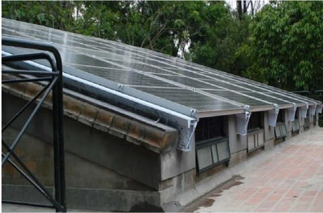
The air channel rows of the BIPV/T installation may be connected in series or in parallel. Simulation results show that the serial connection may result in the highest energy and exergy generations (Agrawal and Tiwari, 2010b).
