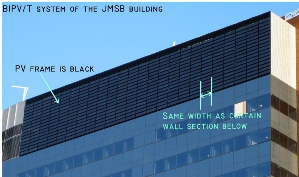
Figure 2.2. The BIPV/T system of the JMSB building
