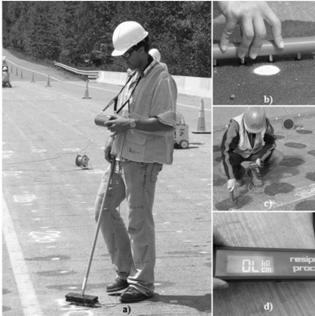
Figure 25. Ponding saturation examples a) Wenner-four probe ; b) Closed view of
