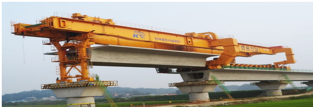
Figure 2-4 Launching Gantry Picking-up the Precast Span (Continental Engineering Corporation, 2006)
