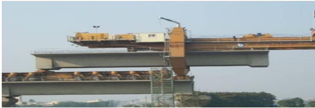
Figure 2-3 Operation of a Launching Gantry (Benaim, 2008)
