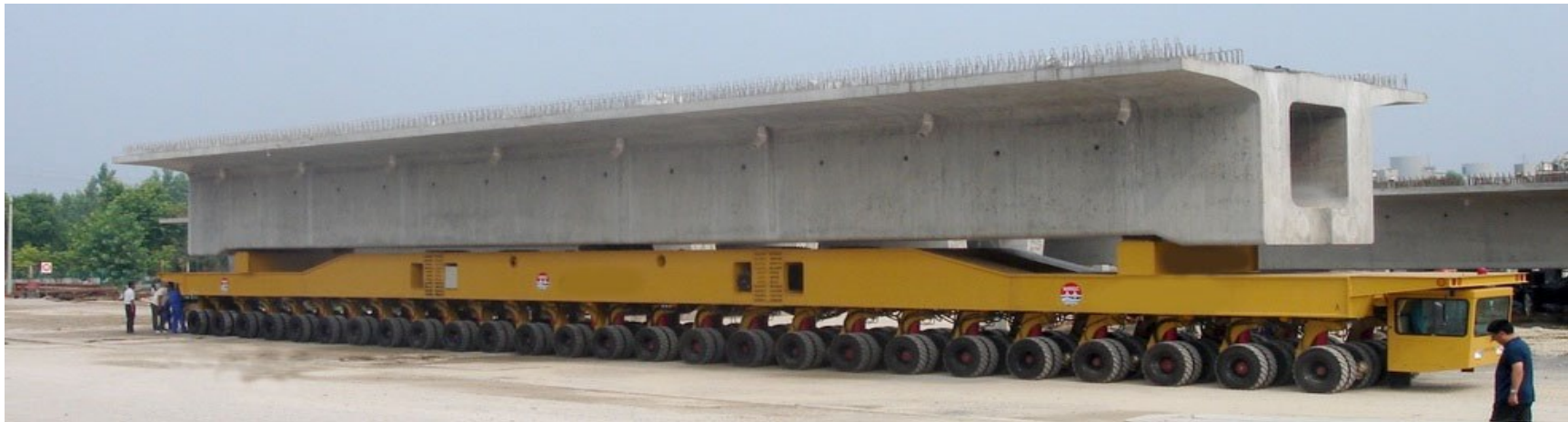
Figure 2-1 Schematic Drawing of Precast Full Span Launching Method (VSL International Ltd., 2013)
