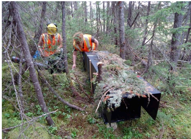
Figure 8: Track box being installed in the forest.
