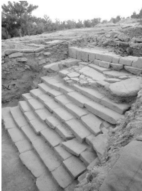
Pl. 29: Doliche - Stone Stairway, Entrance to Dolichenum temenos .
