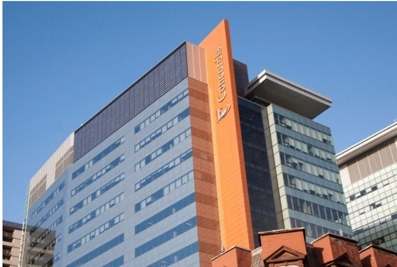
**Figure 2.2:** BIPV/T system of the JMSB Building, Concordia University.
