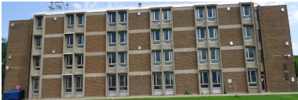
Figure 3.18 : Photo of the south-west façade of HB Building with driving rain gauges
