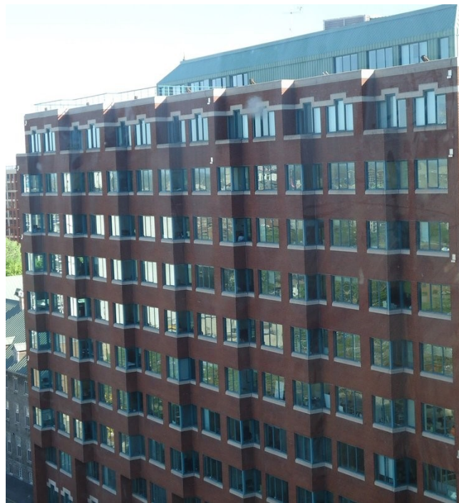
Figure 3.27 : Photo of the north-east façade of FB Building with driving rain gauges
