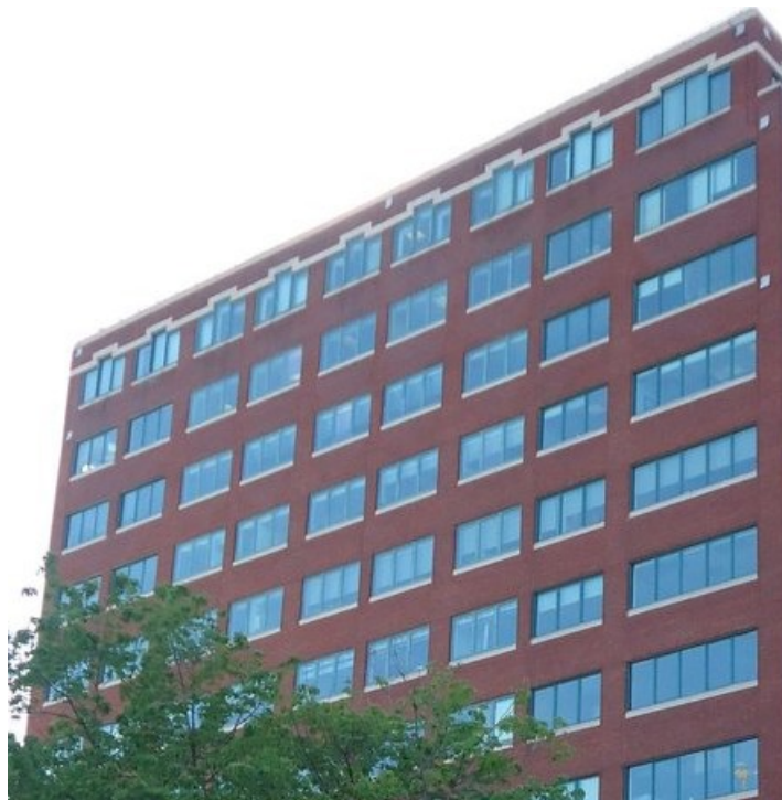
Figure 3.31 : Photo of the south-east façade of FB Building with driving rain gauges
