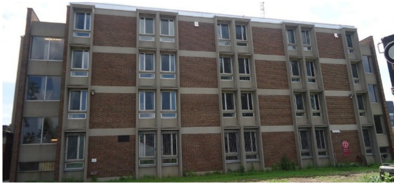
Figure 3.22 : Photo of the north-west façade of HB Building with driving rain gauges
