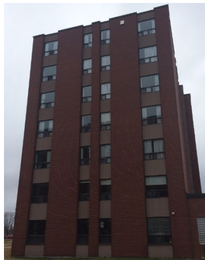
Figure 3.13 : Photo of the north-west façade of McLeod House with driving rain gauges
