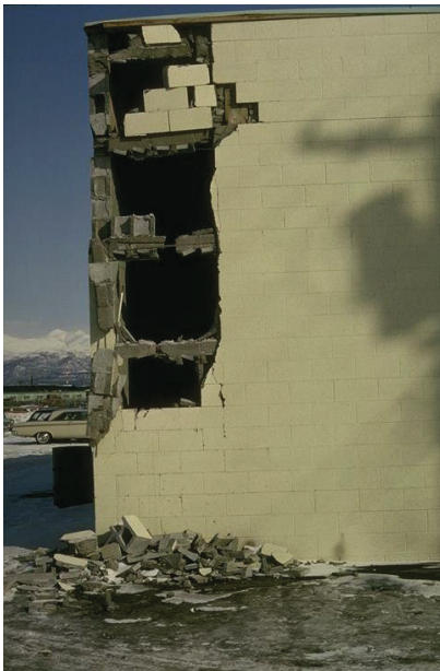
Figure 1.1: Damage to masonry walls due to Alaska earthquake, March 27, 1964 Photos taken by Steinbrugge, Karl V, NISEE, University of California, Berkeley
