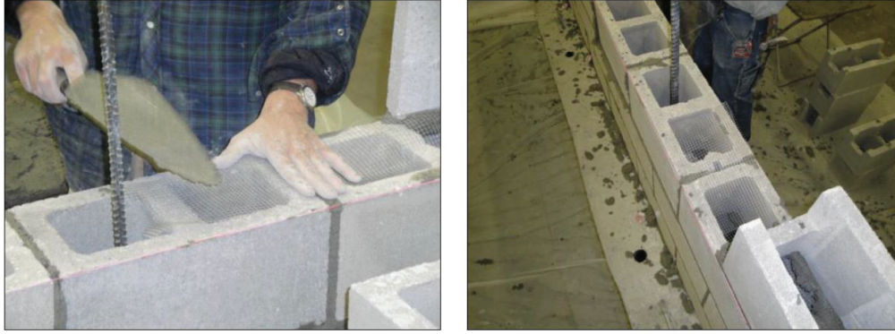
Figure 2.11: Construction of bond beam in partially grouted masonry wall (ElMapruk, 2010)
