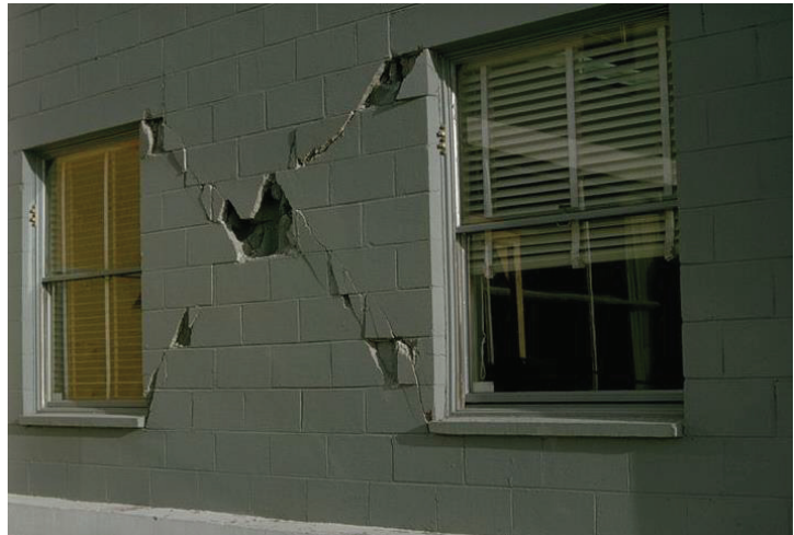
Figure 1.1: Damage to masonry walls due to Alaska earthquake, March 27, 1964 Photos taken by Steinbrugge, Karl V, NISEE, University of California, Berkeley
