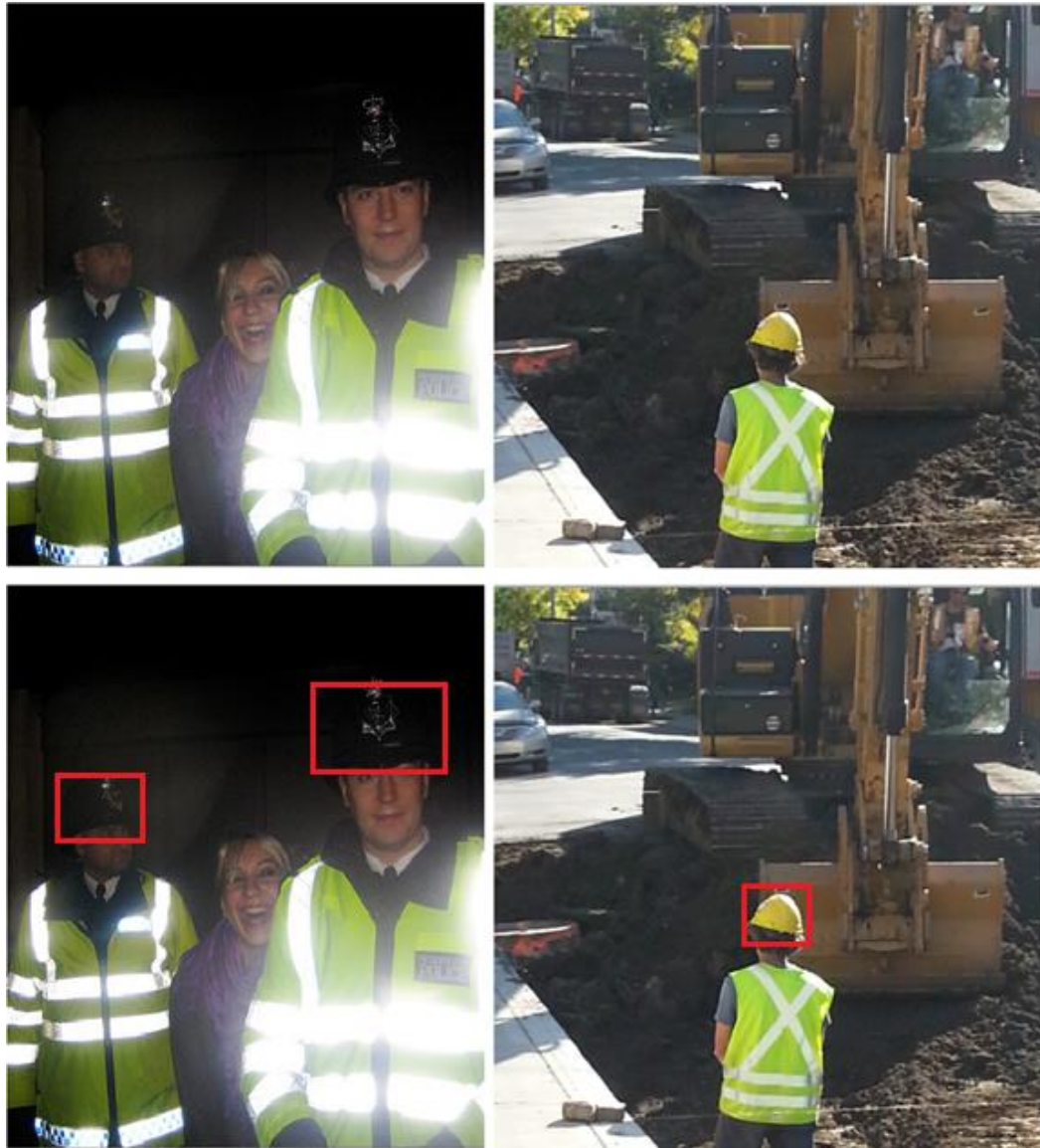
388 Figure 3-9: Darkest image A, and brightest image B with the result of hardhats detection
