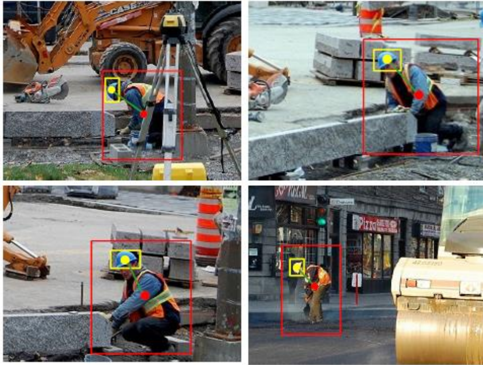
737 Figure 5-1: Potential spatial and geometric relationship between a hardhat and a 738 worker not standing or walking
