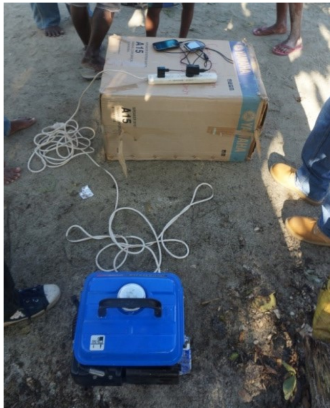
Figure 50: Diesel generator charging mobile phones, Gwou'ulu, September 2014 © Geoffrey & Stephanie Hobbis
