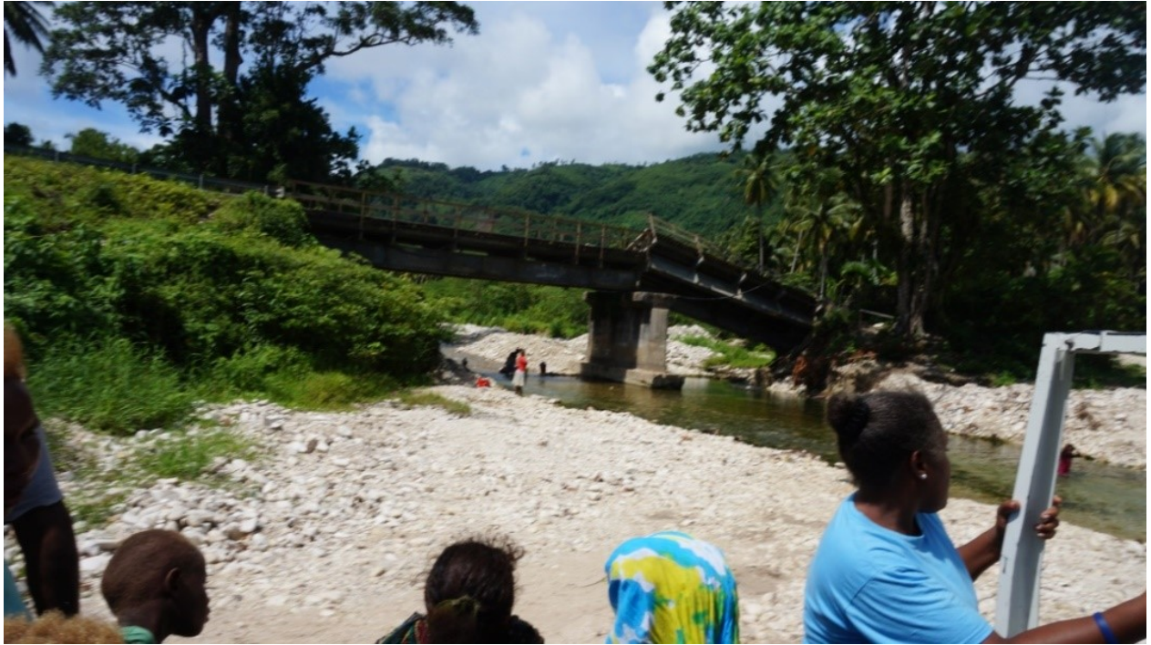
Figure 18: Collapsed bridge, North Road, Malaita, August 2014 © Geoffrey & Stephanie Hobbis
