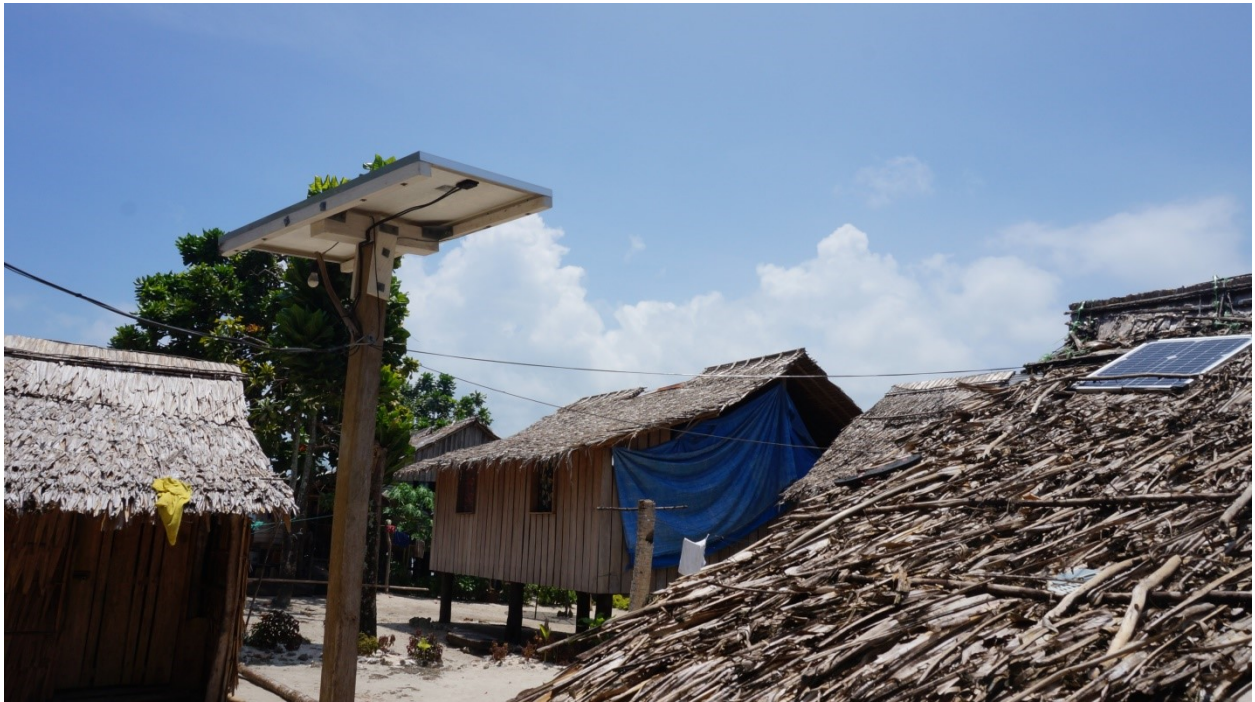
Figure 48: A 120 Watt Solar Power Unit, Gwou'ulu, November 2014 © Geoffrey & Stephanie Hobbis
