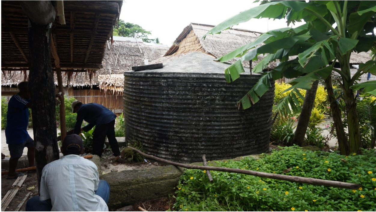
Figure 52: Cement water tank, Gwou'ulu, October 2014 © Geoffrey & Stephanie Hobbis
