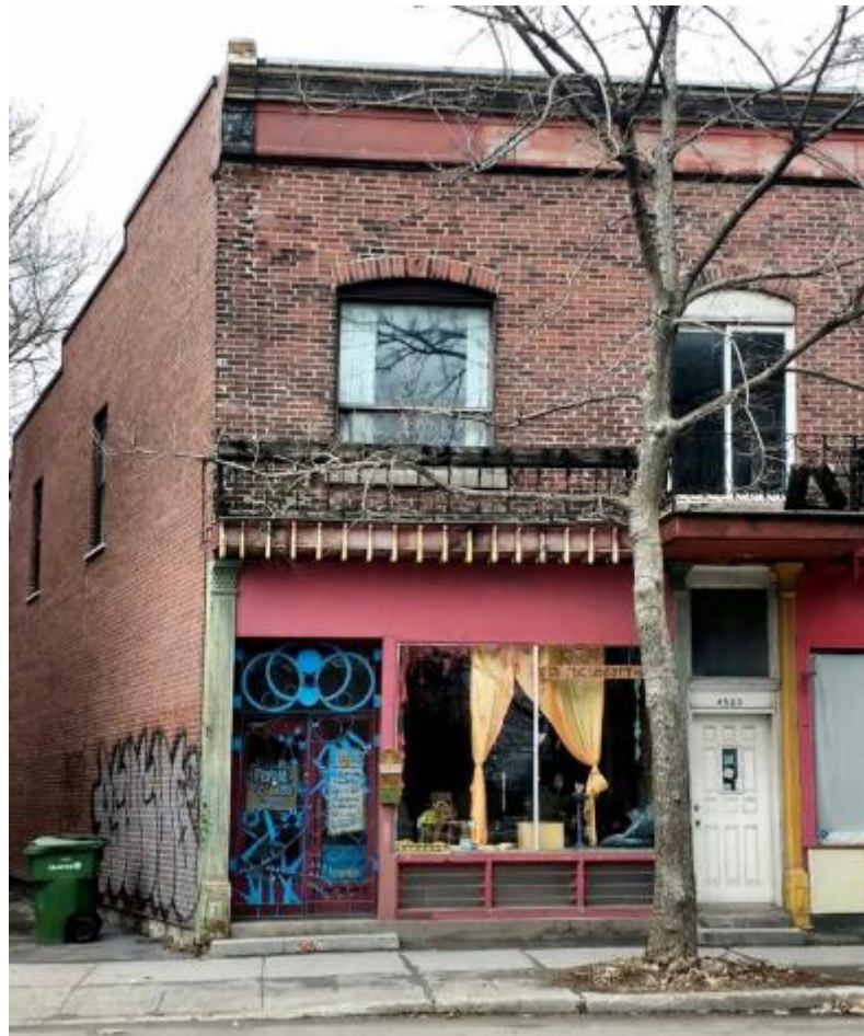
Figure 1. The front façade of La Ruche d'Art: Community Studio and Science Shop Photo: Carmen Despres, 2017
