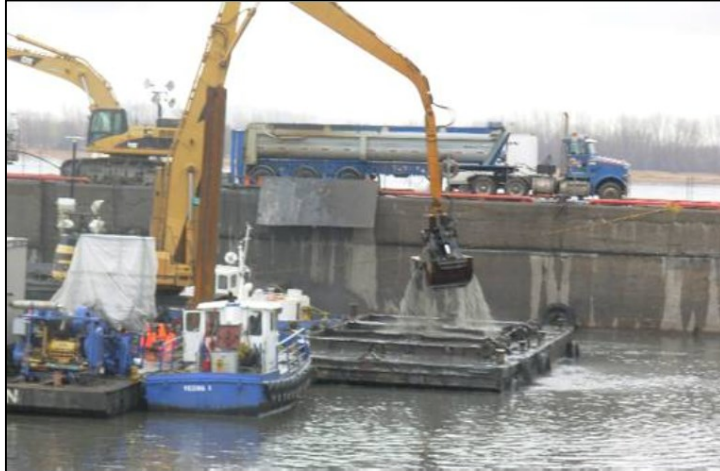
Figure 2.5 Dredging operation by using specialized machinery -Sector 103- Montreal port (Photo: Jacques-Cartier, Environment Canada website)
