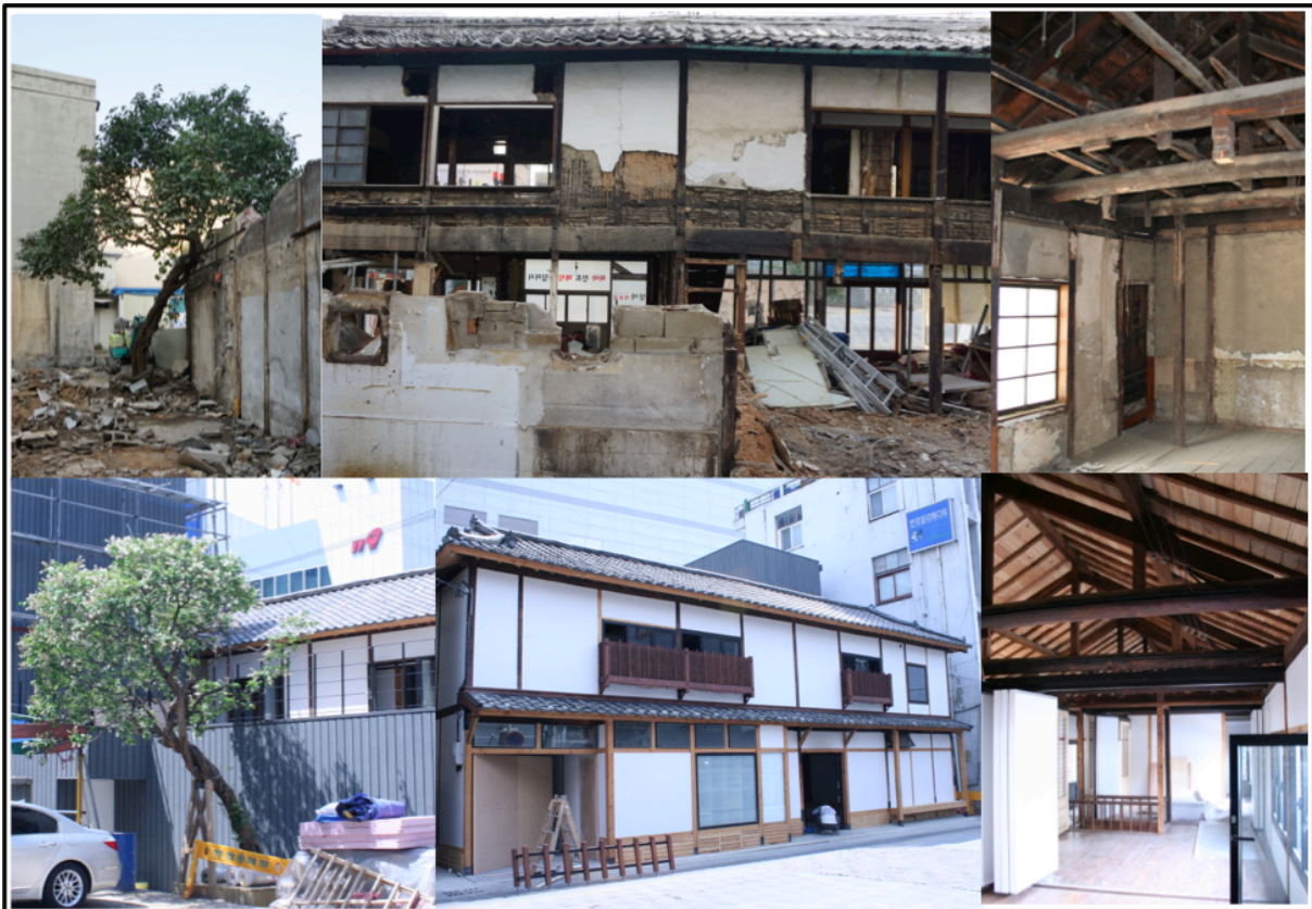
Figure 22. Construction process of the Heeum Museum building
