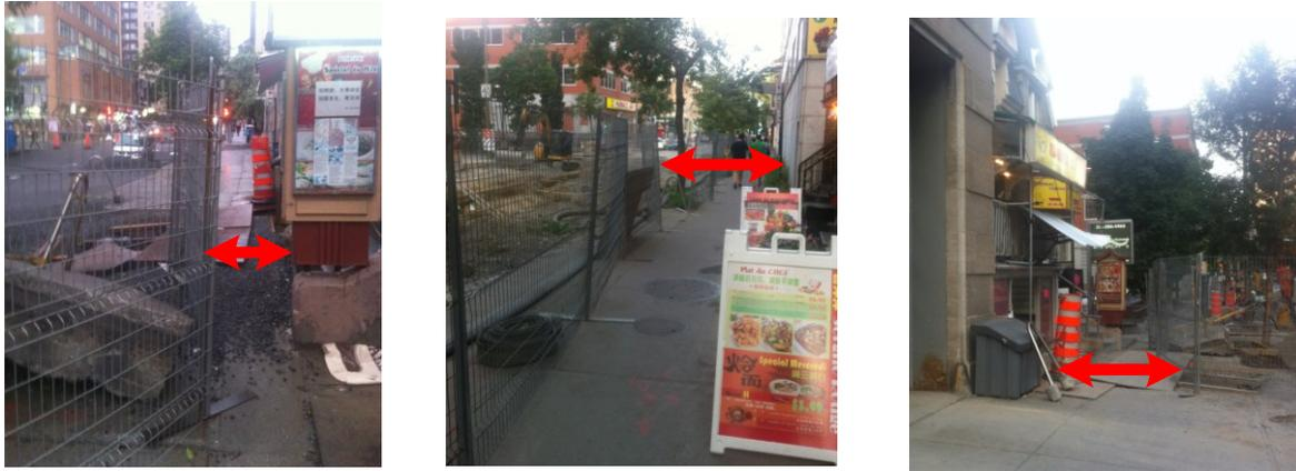
FIGURE J.1: Examples of sidewalk partial closure during works
