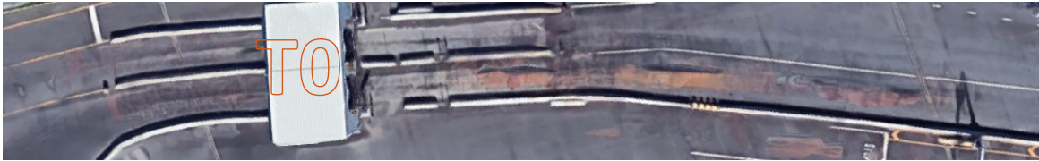
Figure 12 T0 gate entry lanes
