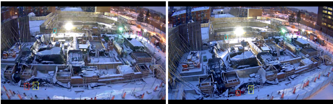
Figure 4.11 Workers matching at night
