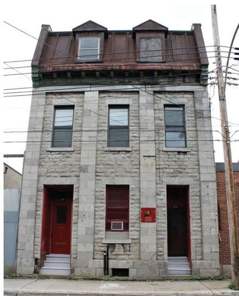
Fig. 5. Centaur Theatre rehearsal space and former Griffintown police station. September 2010. Photo by author.
