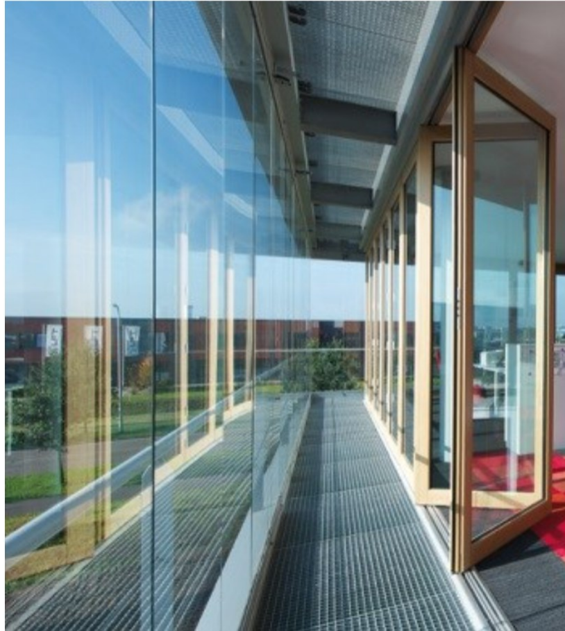
Figure 1. An example of DFS in a new office building in the Netherlands [ https://facadeworld.com/2014/03/15/solarlux-nijverdal/ ]
