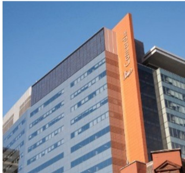
Figure 3. BIPV/T demonstration project in a Concordia University building in Montreal. (Athienitis et al. 2011)
