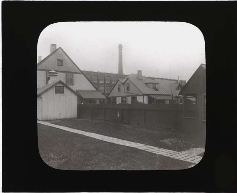
Fig. 23a. "Worker houses and gardens before landscaping." (Photography by Frances Benjamin Johnston, National Cash Register, Dayton, Ohio [ca. 1896]. Glass lantern slide. Courtesy of Library of Congress Prints and Photographs Division Washington, D.C.)
