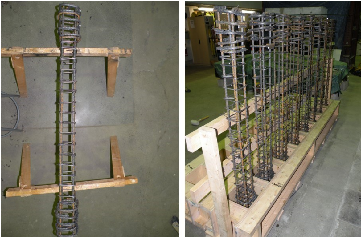
Figure A.14 Assembling the reinforcement steel cages.
