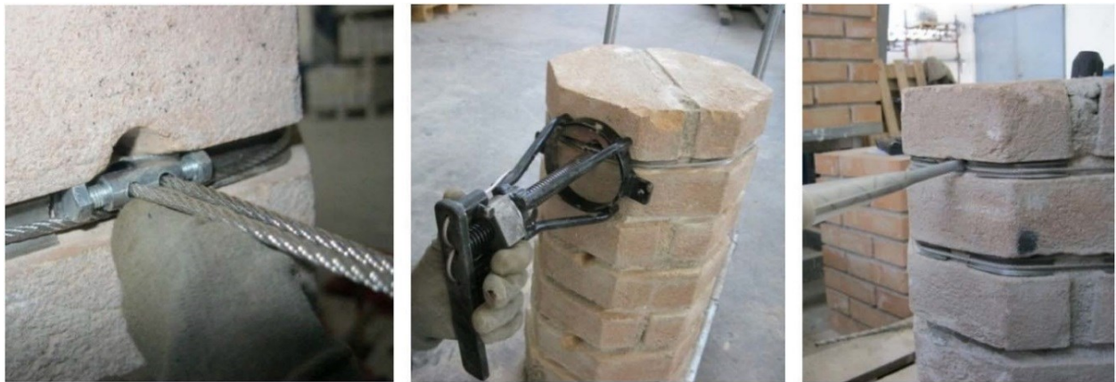
Figure 2.4 Hooping solid clay bricks masonry with pre-tensioned steel cords (Borri et al., 2013).
