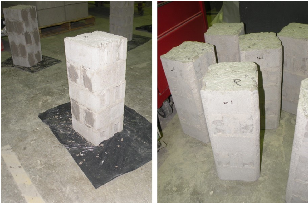
Figure A.9 Filling the flanged ends of the concrete block units with a repair mortar.
