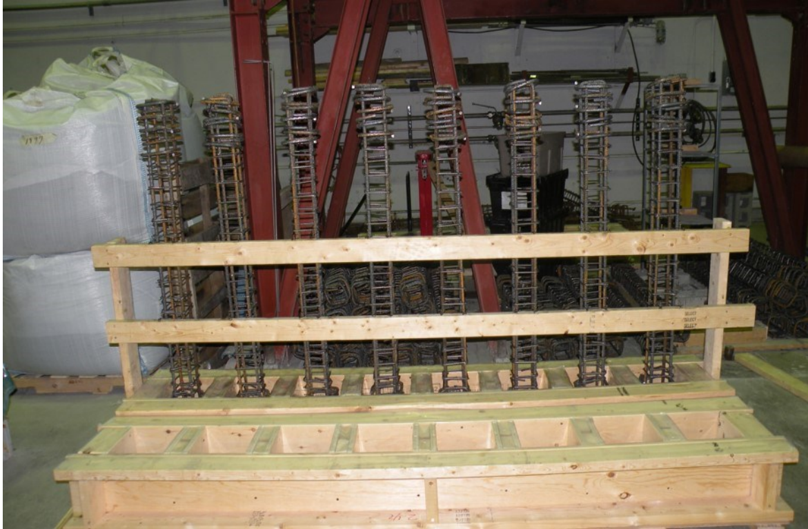
Figure A.15 Wooden formwork for the bottom concrete footings.
