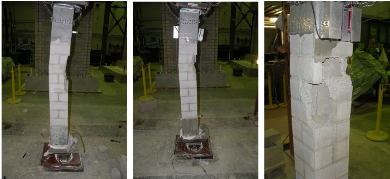
Figure C.24 Failure modes at the end of the eccentric tests for L0-e40.
