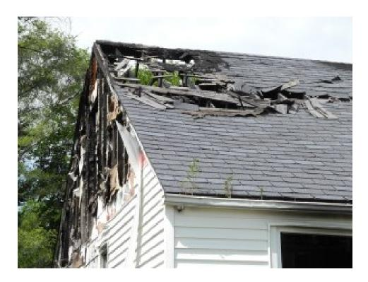
Figure 1-2: Large roof damage of gabled roof building caused by heavy winds in Chicago's Park, April 2016 (http://www.skylinenewspaper.com/wind-storm-rips-roof-from-apartment-building/).
