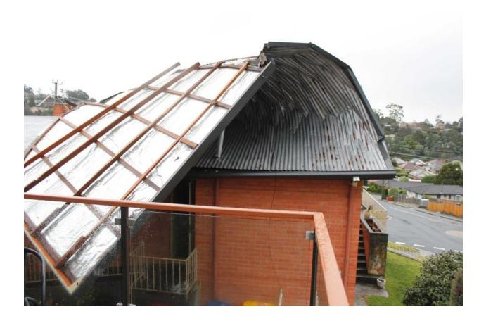
Figure 1-1: Roof damage of a new building due to a wind storm in Tasmania, April 2017 (http://www.abc.net.au/news/2017-04-27/the-roof-peeled-back-from-a-house-in-kings-meadows/8475332).
