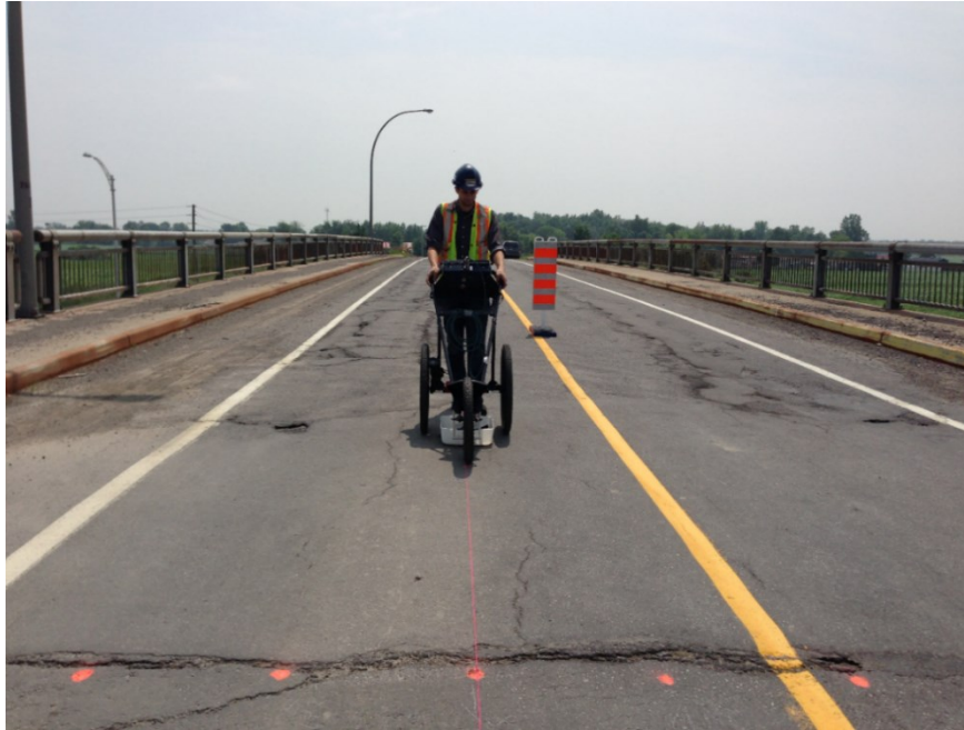
Figure 4.4: Bridge A deck scanning with GPR tool
