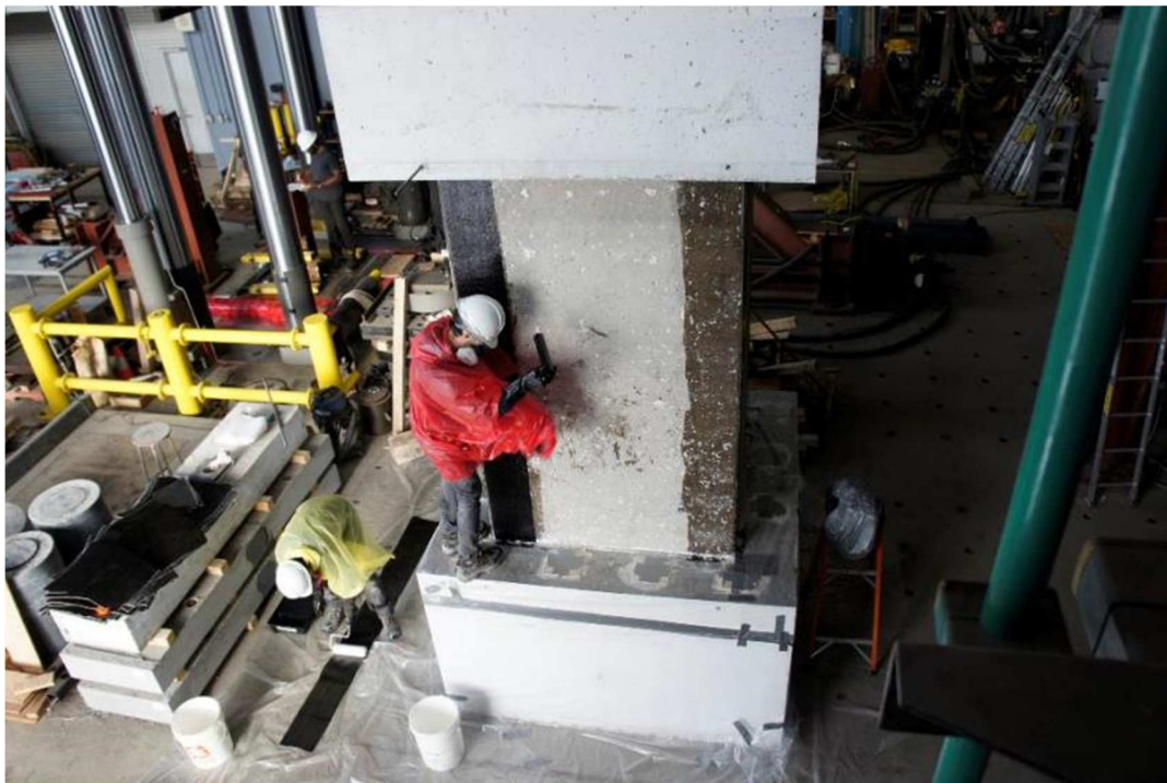
Fig. 6.15. Manual saturation and installation of vertical strips
