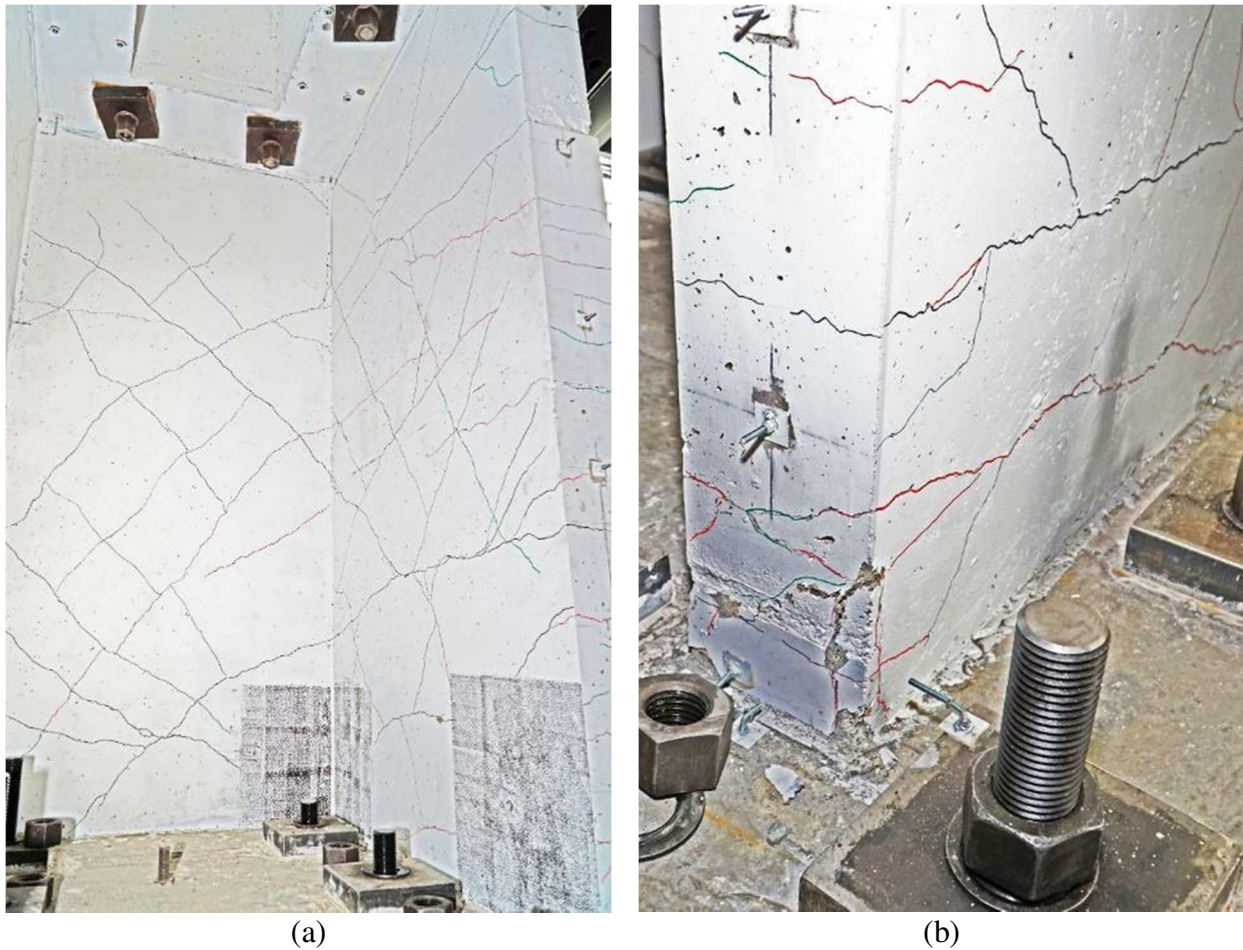
Fig. 6.7. Crack patterns observed at the end of test on Original wall specimen: a) Inside the core wall, b) North-East corner (Mehmachi and Bouaanani, 2018)
