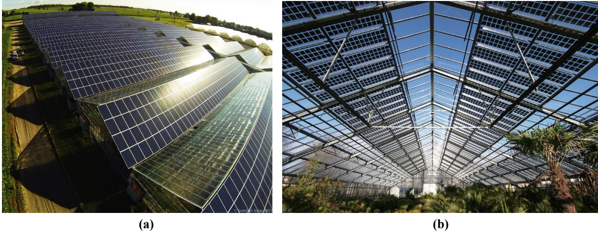
Figure 2.9: (a) Opaque PV module employed on the south-facing greenhouse roof (Enphase, 2015); (b) STPV modules integrated into a greenhouse roof (Agrithermic, 2018).
