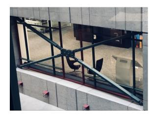
Figure 1-2 Pall Friction dampers installed in the Webster Library of Concordia University,
