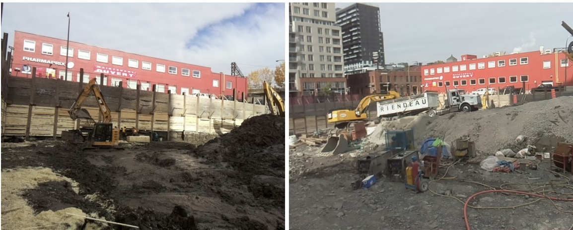
Figure 35 Image samples of Amati construction site
