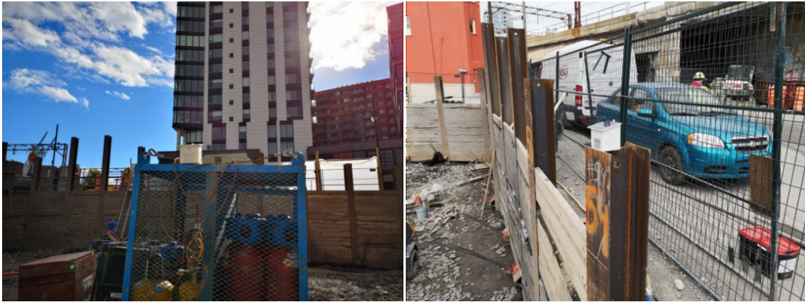
Figure 48 Placement of the monitoring system
