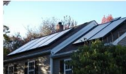
Residence, Halifax, Nova Scotia, Canada 6 - G32-P Solar collectors Solar Radiant Floor Heating, Solar Domestic Hot Water
