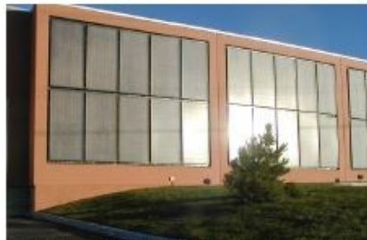
Thermo Dynamics Ltd., Dartmouth, Nova Scotia, Canada 30 - G32-P Solar collectors Solar Radiant Floor Heating
