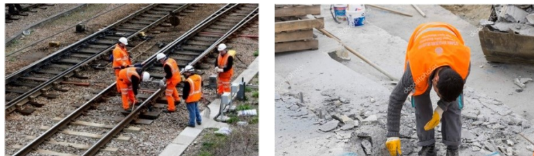
(a) Workers with hardhat and safety vests (b) Worker without hardhat
