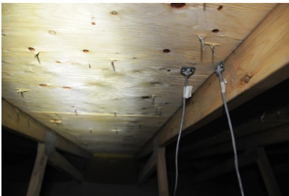
Figure 3-13. No signs of moisture on building materials. Roofing nails not rusted.
