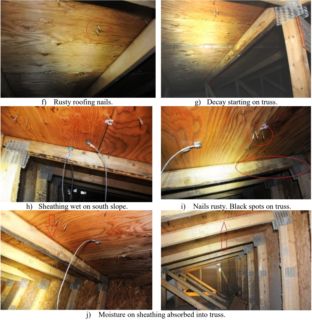
Figure 3-16. Field observation of un-ventilated attic of House III (SIP House).
