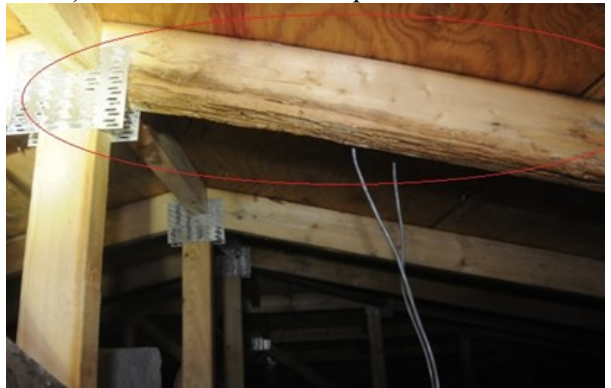
c) Decay of truss occurring above hatch location.
