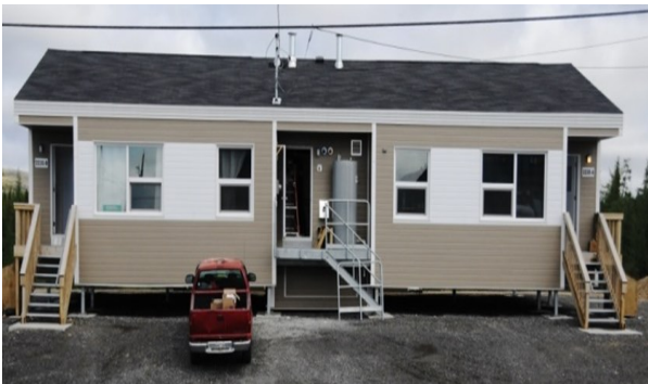
a) House I (KMHB House).
