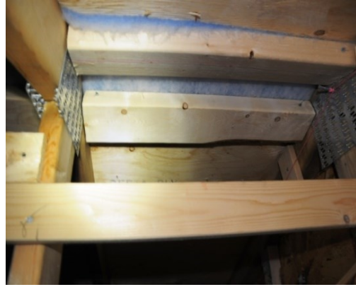
Figure 3-12. Filter membrane installed at ridge vent.
