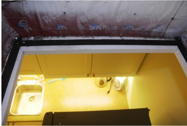
Figure 3-15. Weather stripping installed on opening trim in all units.
