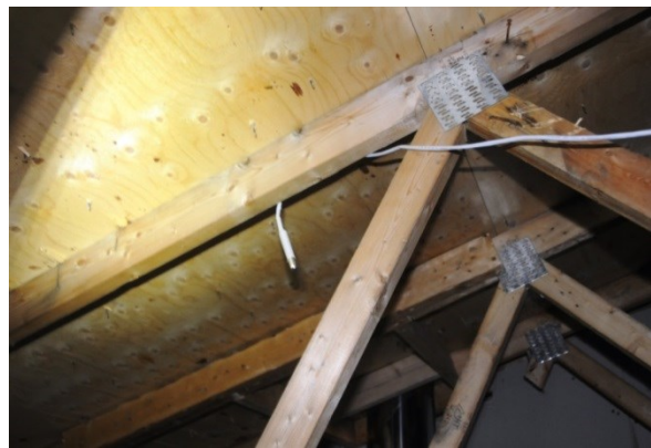
Figure 3-13. No signs of moisture on building materials. Roofing nails not rusted.
