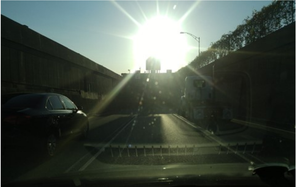
Figure 2.2: A photo taken by D. Sun at approximately the safe stopping distance from the tunnel portal at the Louis-Hippolyte-La Fontaine tunnel [2].
