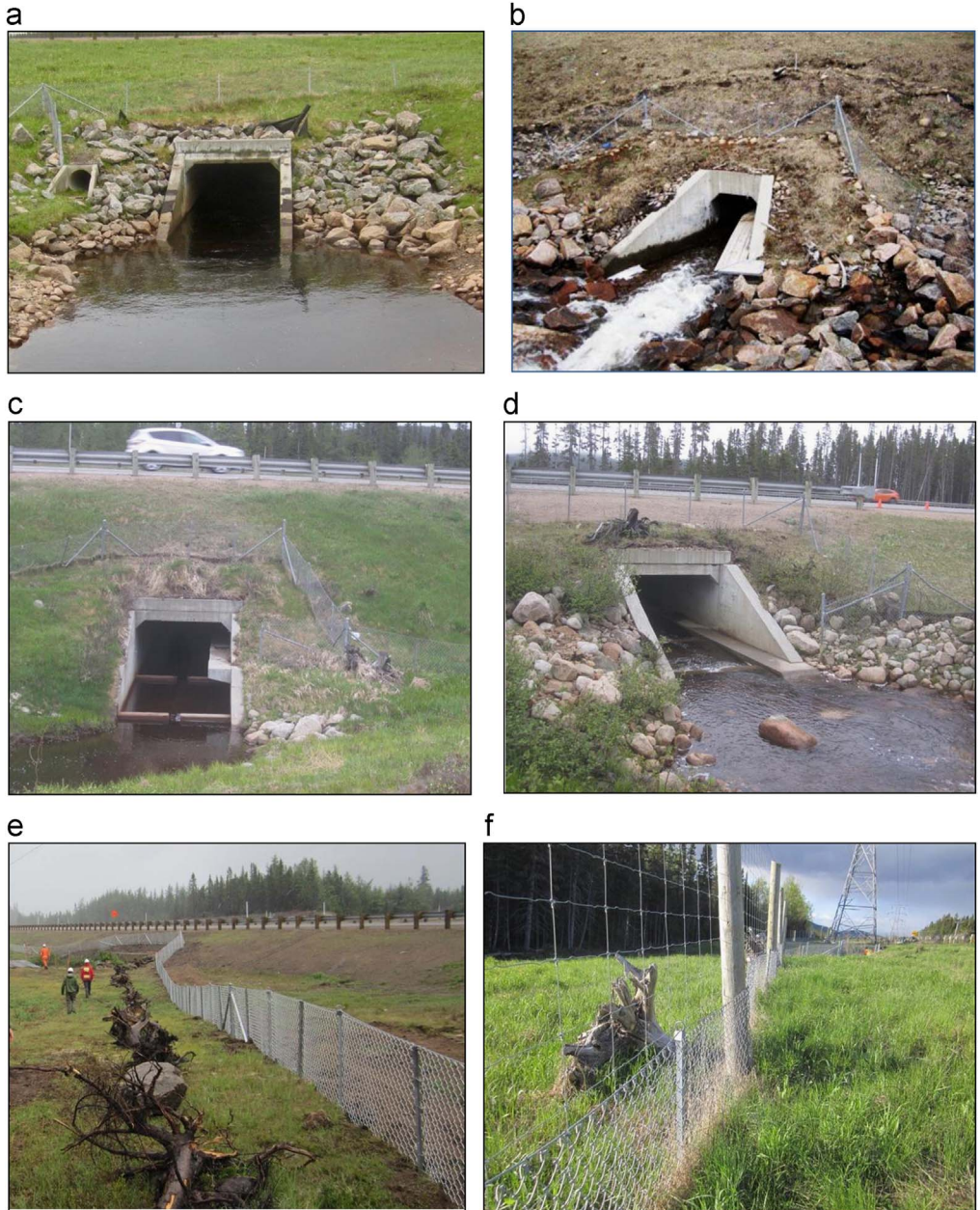
Fig. 2. The four types of wildlife underpasses designed for small and medium-sized mammals and the two types of fences along Highway 175: (a) pipe culvert or round concrete culvert (on the left next to the water culvert; n = 6 ), (b) box culvert with a wooden ledge ( n = 4 ), (c) box culvert with a concrete ledge ( n = 7 ), (d) box culvert with a concrete walkway ( n = 1 ), (e) fence for medium-sized mammals, and (f) combined fencing for large mammals (upper half) and medium-sized mammals (lower half) (photo credit: Concordia University).
