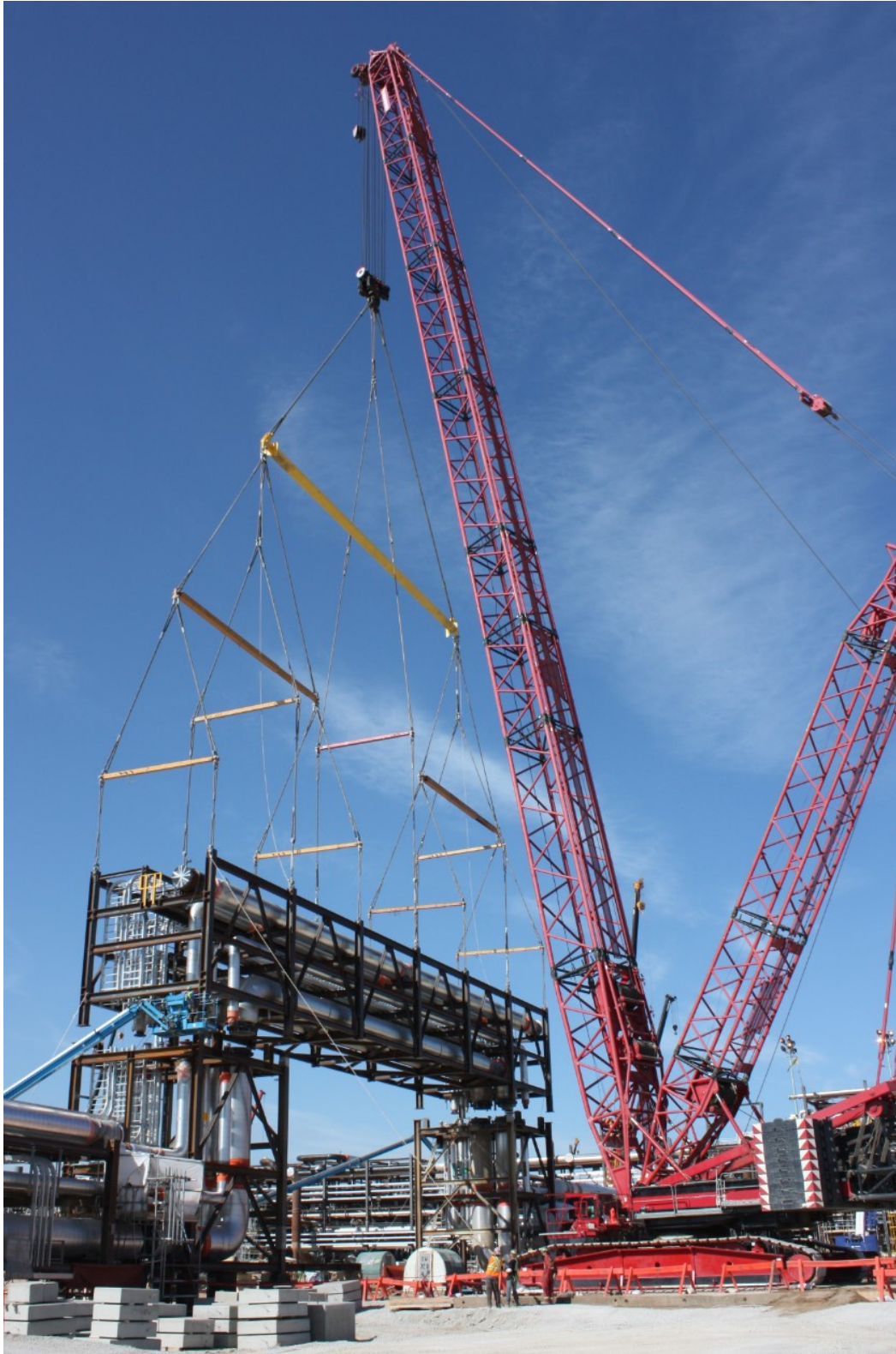
Fig. 4. Lifting an industrial 12-point pick module
