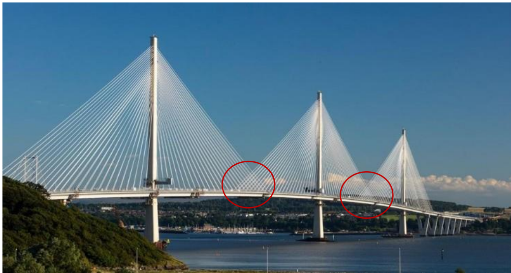
Figure 2.11 Photo of Queensferry Crossing Bridge, Scotland (Source: Transport Scotland).
