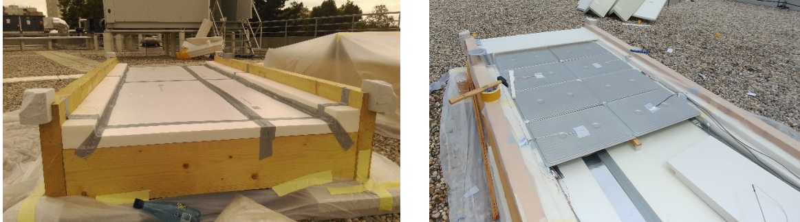
Figure 29. Main construction elements (wood and polystyrene sections) for both prototypes
