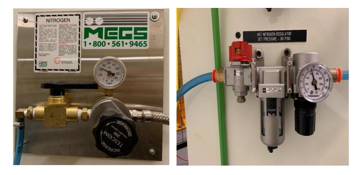
**Figure 22.** Nitrogen supply line (Left); HGT nitrogen regulator (Right)
