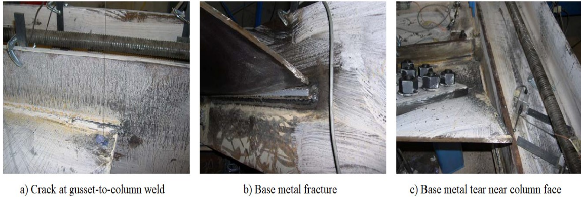
Figure 2.9 Experimental brace-to-frame connection failure a) Crack at gusset-to-column weld b) Base metal fracture c) Base metal tear near column face (Kotulka, 2007)
