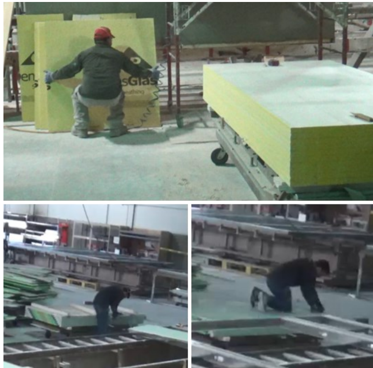
Fig. 11. Existing drywall preparation station
